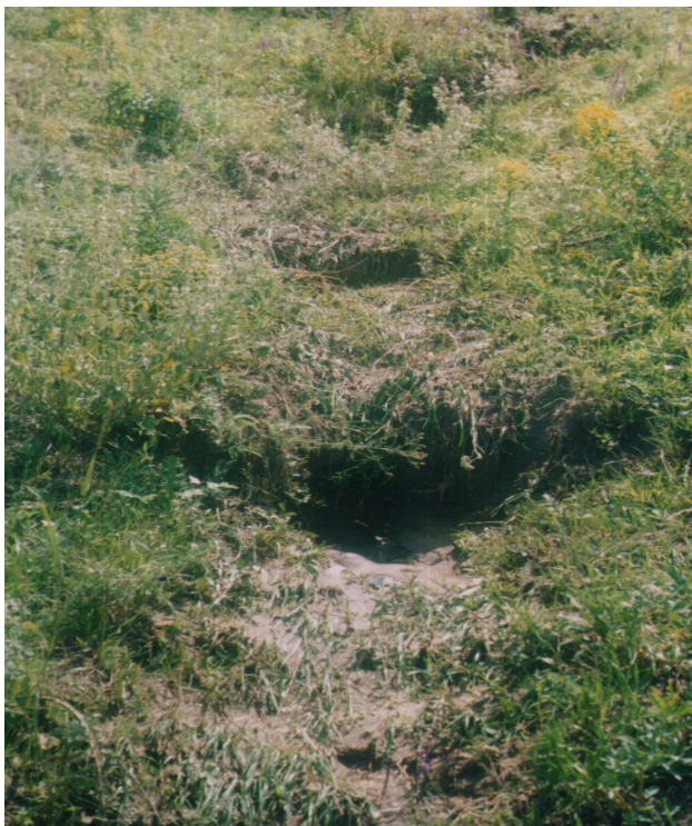
Figure 2. Alternation of places of loss in the bottom part of a slope on rangelands a slope
