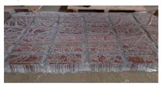
Figure 3. Curing with plastic sheet
